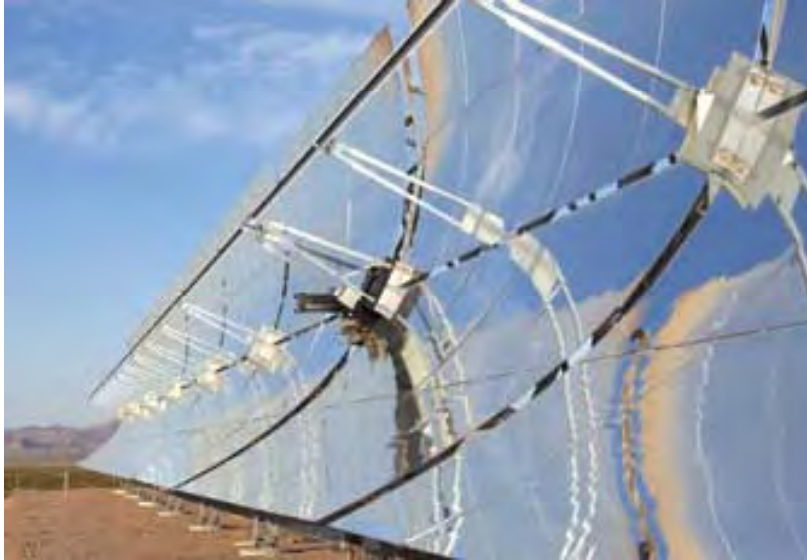
Parabolic Trough Systems
